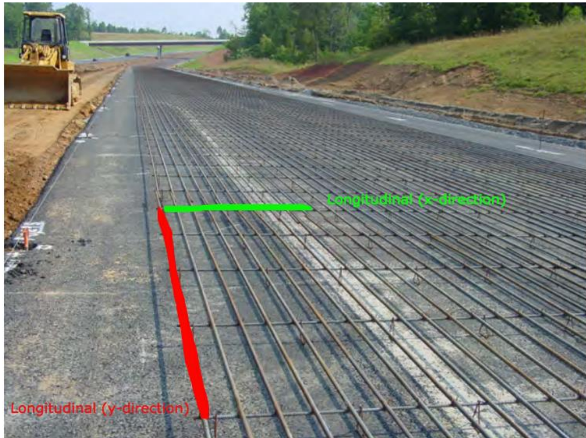
Figure 12: Steel reinforcement for concrete pavements, x-, y- direction
