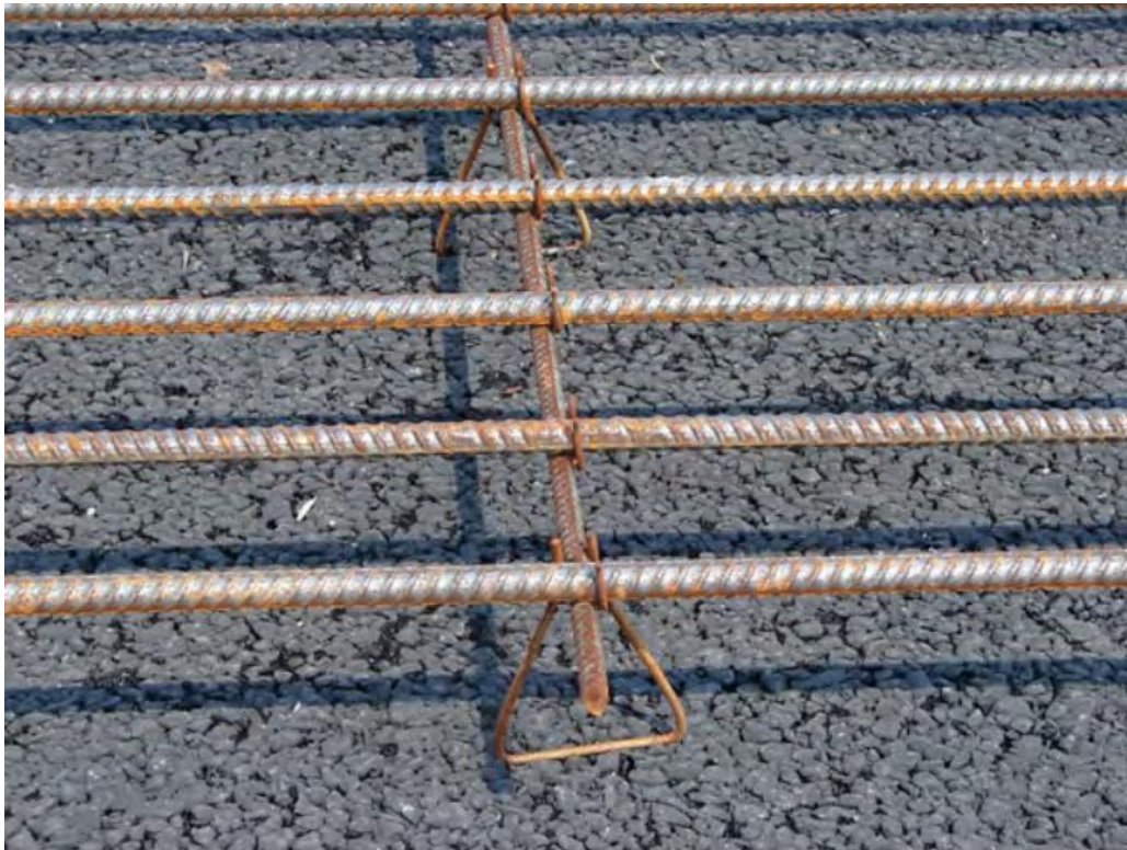
Figure 14: Steel dowel support for distance to bottom
