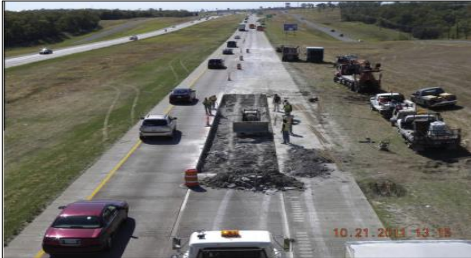
Figure 2: FDR performed in Texas, USA, where the road is improved with two layers of steel reinforcement in an effort to prevent future cracking (Chen, et al., 2014)
