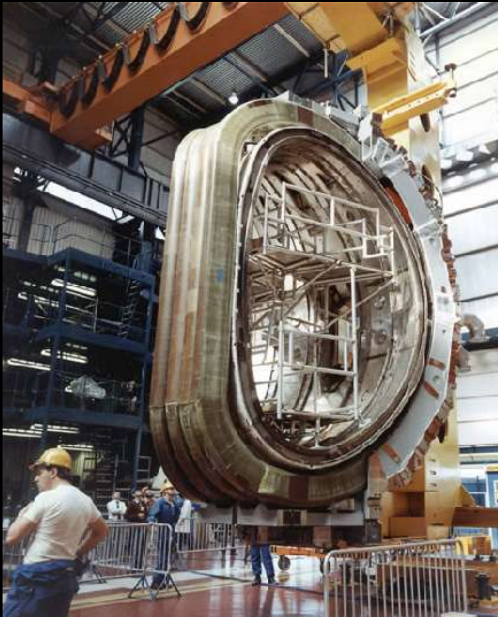
An octant section of JET's torus, held in a C-frame, 1982
