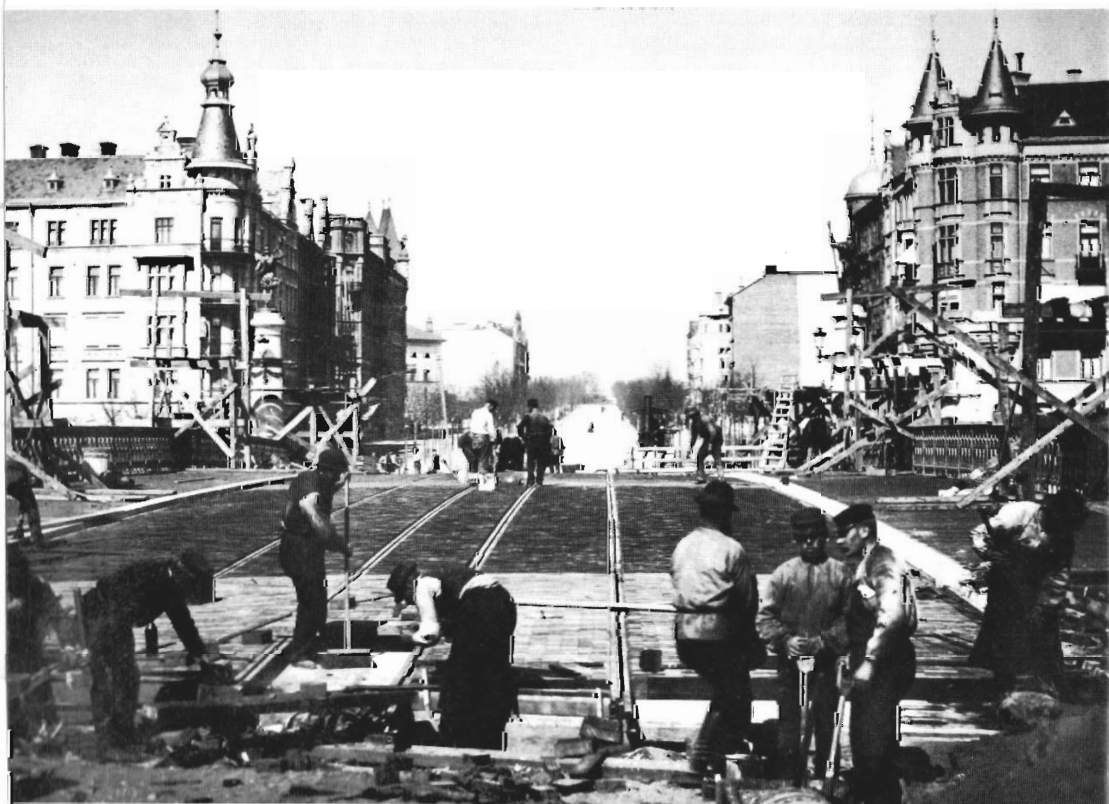
Paving Djurgård Bridge with wooden blocks during construction work on the tramway. In the distance can be seen the wide esplanade of Narvavägen, not yet fully developed. 1897.
