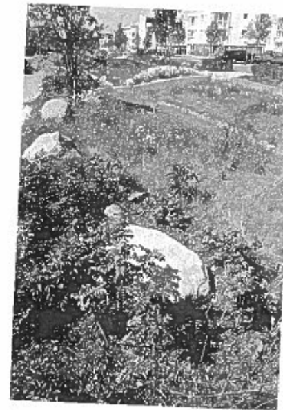
Figure 11 Natural stormwater collection system at the Kronsberg Ecological District, in Hannover, Germany. Source: Photograph by Timothy Beatley.
